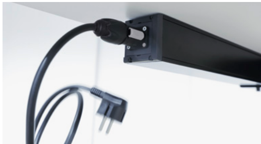
The supply lead is pushed in...
